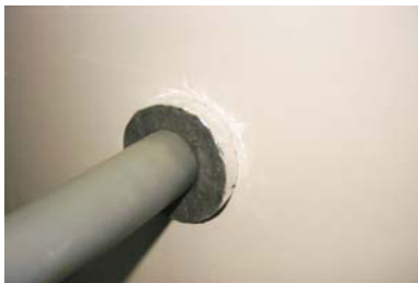
Fire sleeve fitted into wall
